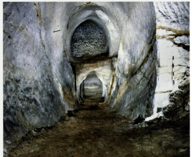
Reigate Lodge North mine in June 1986: mining on two levels separated by an iron-cemented 'carstone' band can be seen. Photo Nick Catford
